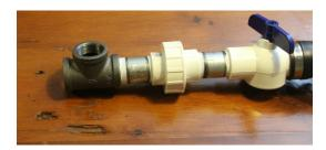
7. On the two remaining sections of the tee, screw 1-1/4" pipe nipples securely.
