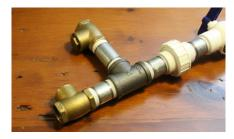
10. From this check valve, install another pipe nipple.
