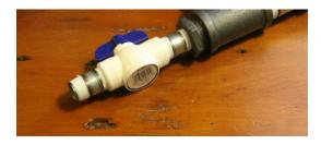
21. Make sure that the 3/4" union is connected together. Screw it onto the 3/4" pipe nipple.
