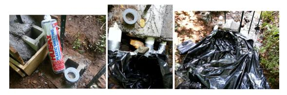
Once the plastic was secured to the pipes I placed the other end into the creek so that water started to run onto it. I had to take several rocks to place on the plastic to keep it from floating up and washing out. The tape held well and the water started to flow out of the pipes.
