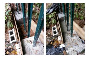
Once the concrete had finished doing, whatever concrete does as it sets up, I moved the wooden form and set it on the hill. The water seems to have stopped flowing from the creek and was now coming out of the pipes. That was just what I wanted. Now that the creek was officially dammed I needed to finish building the wall up.
