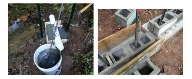
When I set two blocks down I had to go back and pour concrete between them to fill the gaps and to secure the blocks together. Because I had only purchased one set of wood for the form I could only set up three blocks at a time. This was alright though because in this early stage of my concrete knowledge I did not need to do more than 2 bags. I
